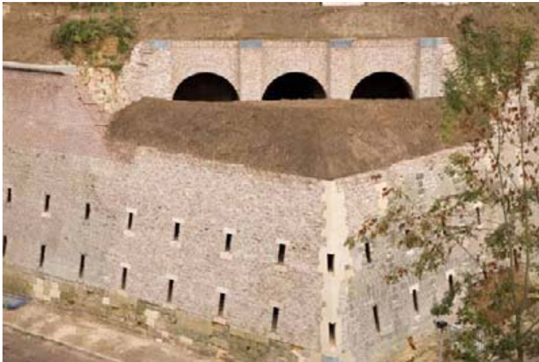
Fort St. Pieter na restauratie in 2006.
